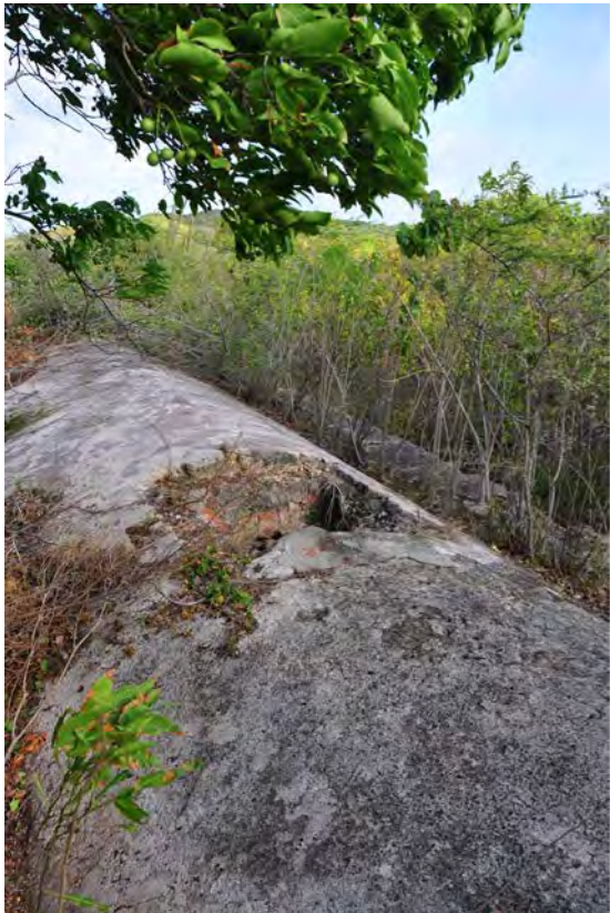
Figure 44. Cistern at the Artillery Complex.
