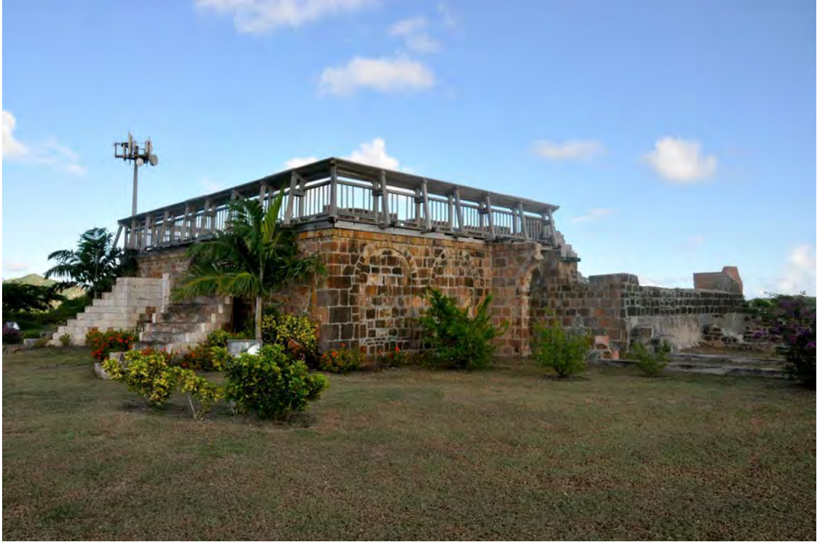
Figure 30. Stabilized ruins of Dow's Hill Governor's Residence.
