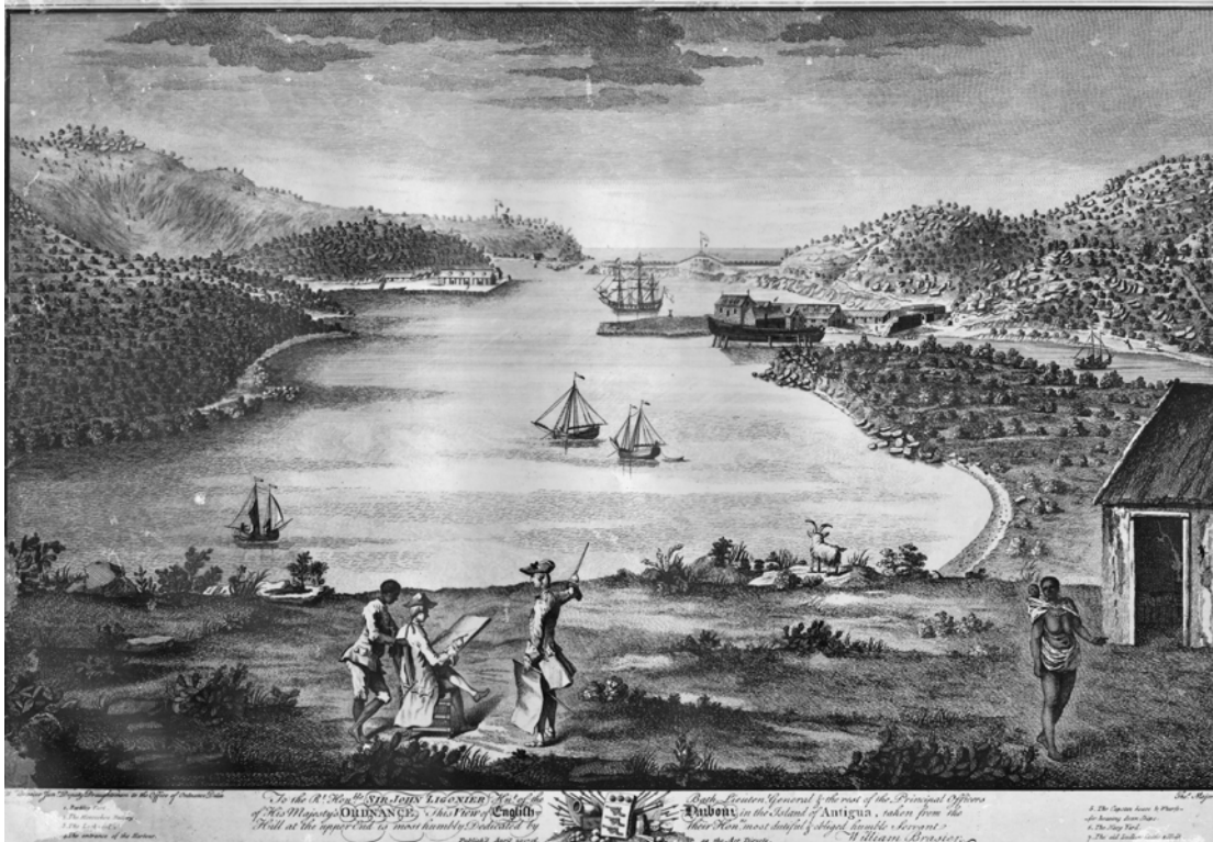
Figure 83. View of Ordnance Bay in the foreground looking towards the Dockyard.
