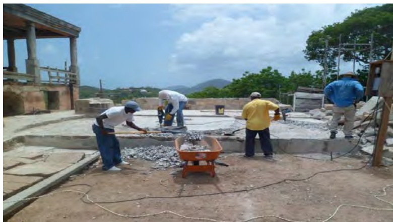
Restorative Work at Clarence House
