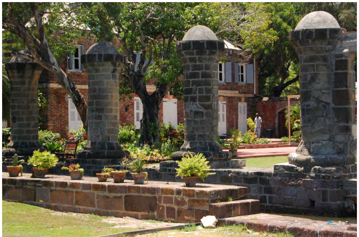
Figure 7. The Sail Loft Columns with the Engineers House in the Background
