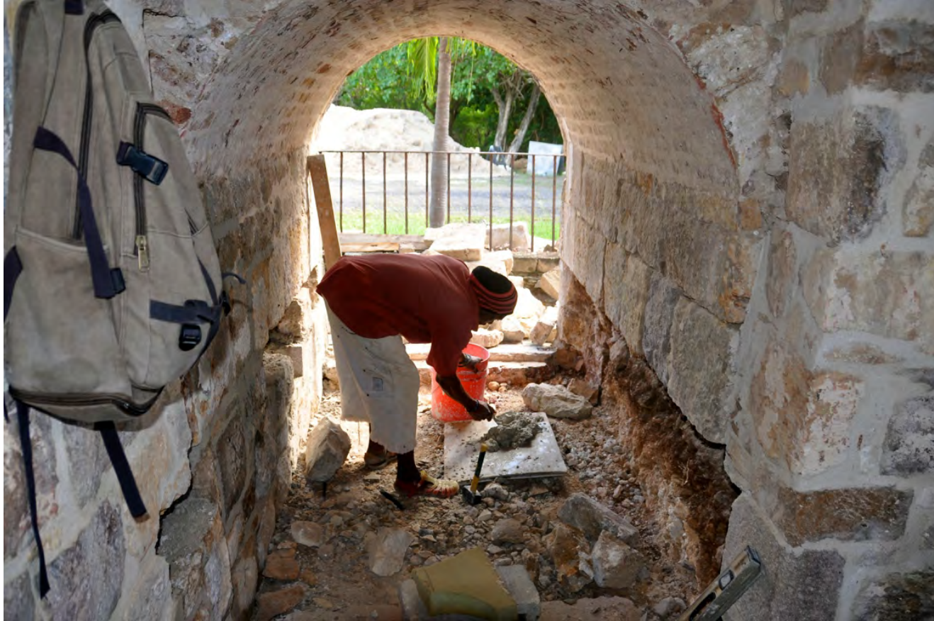
STONE MASONS AT WORK ON THE CLARENCE HOUSE RESTORATION PROJECT
