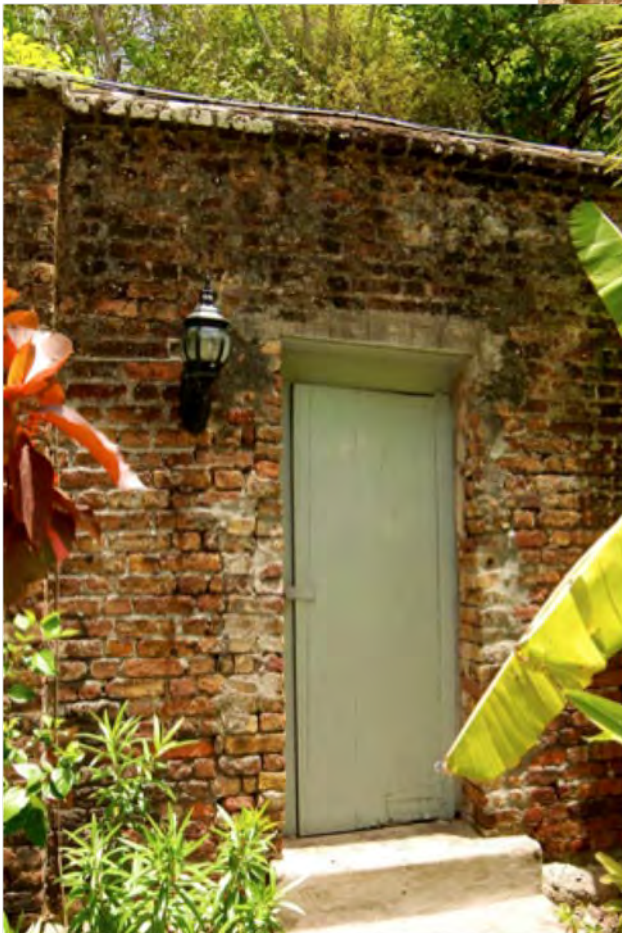
Small Entry Door into Engineers House area
