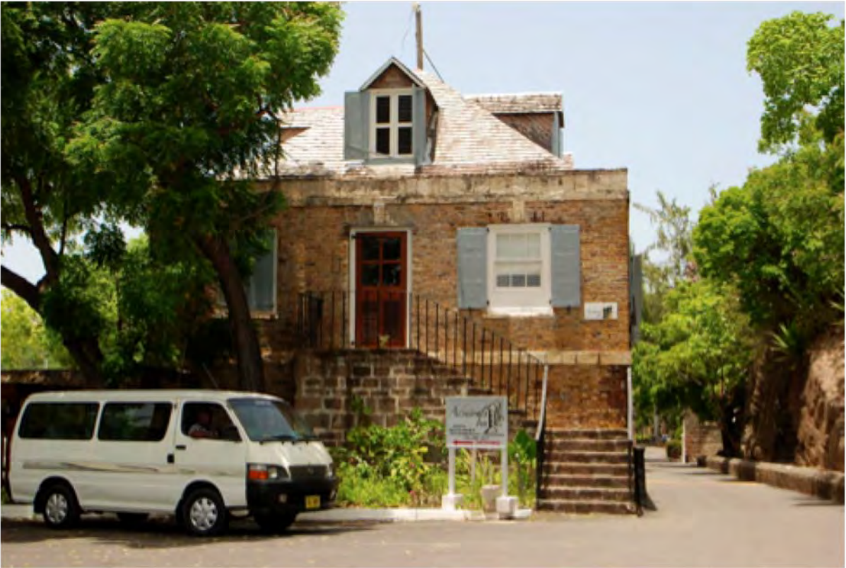
West view of the Engineers Building
