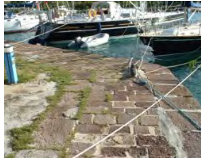
Section of old seawall
