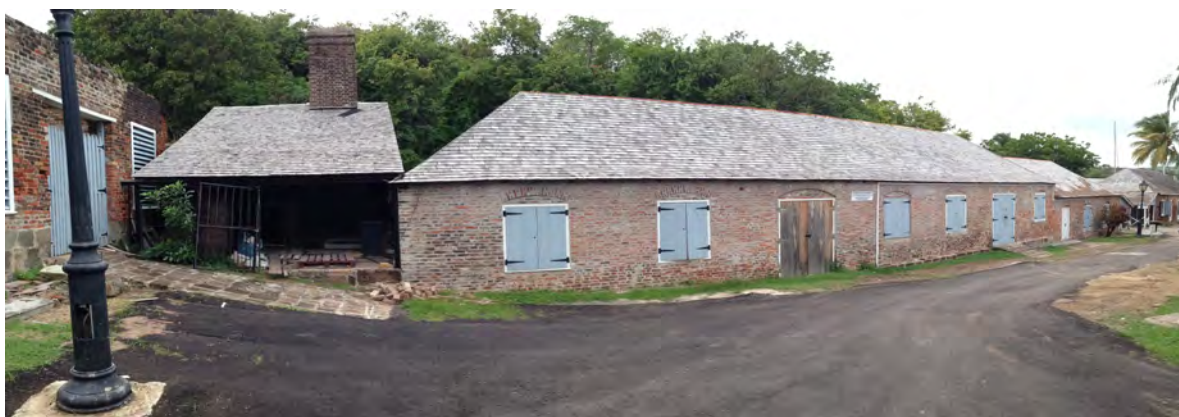
Figure 15. The Guard Station and Engineer's Storage and Workshop
