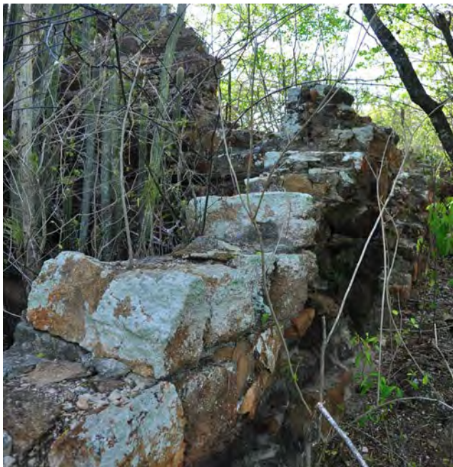
Figure 34. Ruins on north side of Ridge.
