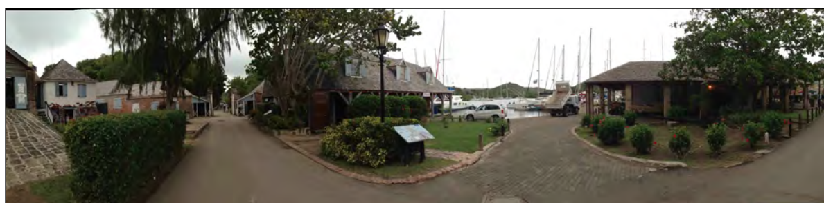
Figure 11. Entry Gate and Mast Shed area of the Dockyard.
