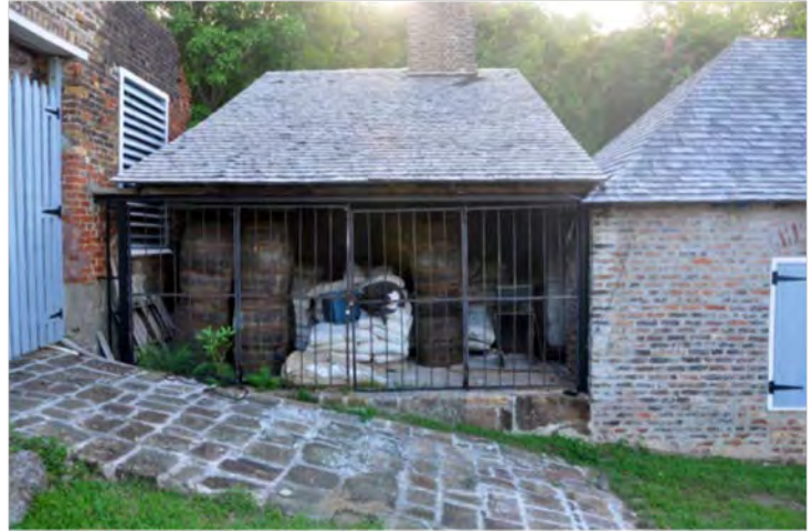
Newer Blacksmiths work area with Chimney
