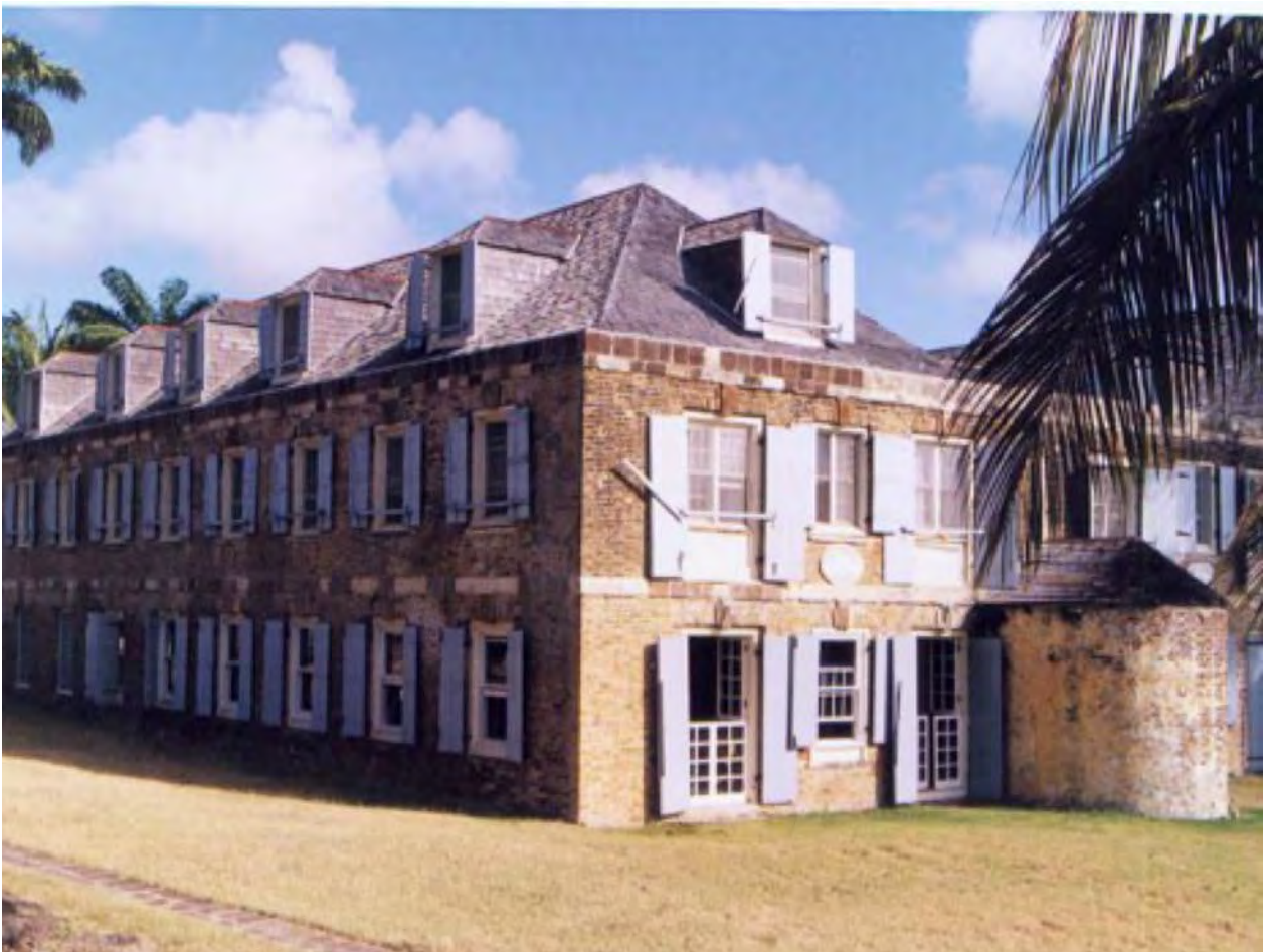
East elevation of Copper and Lumber Store
