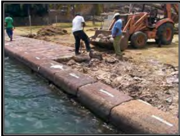
Removal of the old stone seawall.
