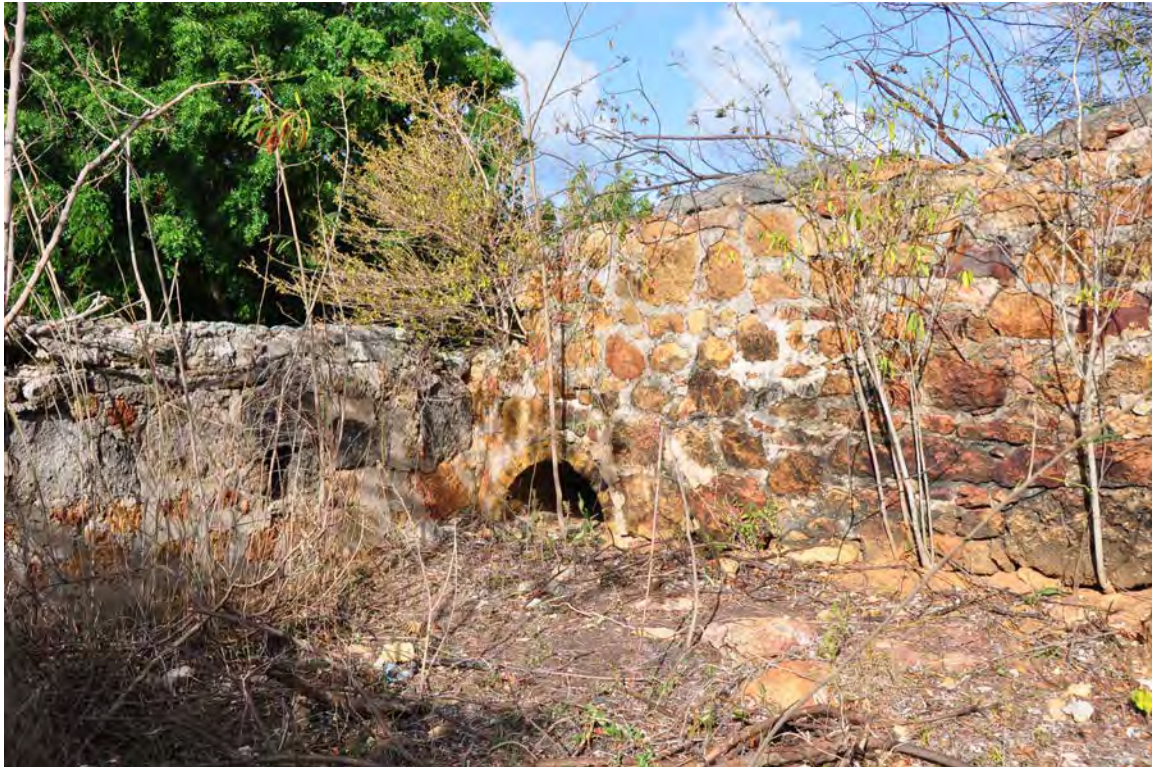
Figure 25. Catchment pond with brick in flow channel.
