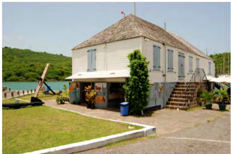
Pay Office South West elevation
