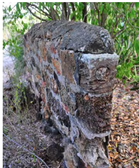
Figure 36. Enclosing wall, possibly of General Stores area.
