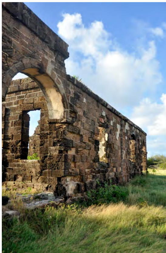
Figure 61. Ruin of Officers Quarters at Block House Complex
