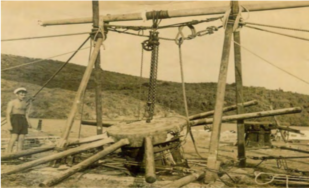
Figure 45. Capstan being removed for restoration 1950
