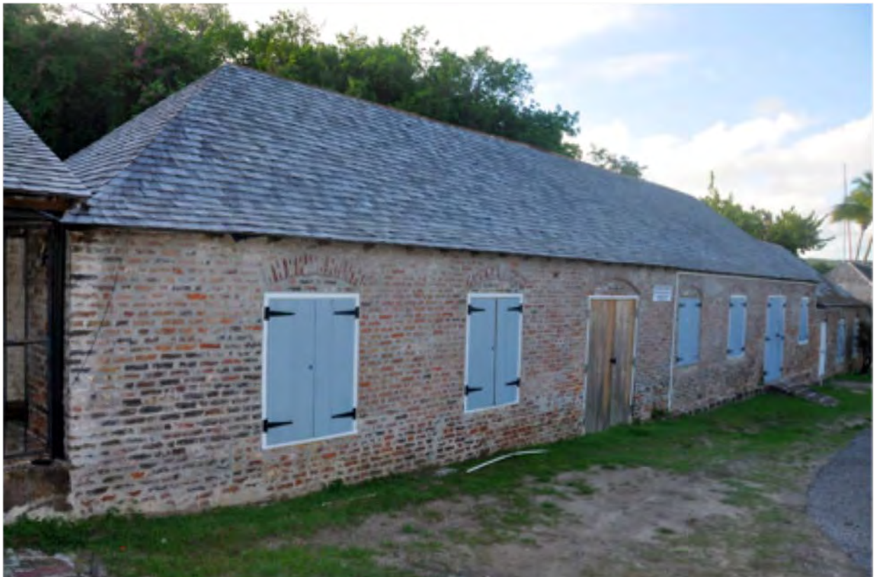
The Engineers workshop
