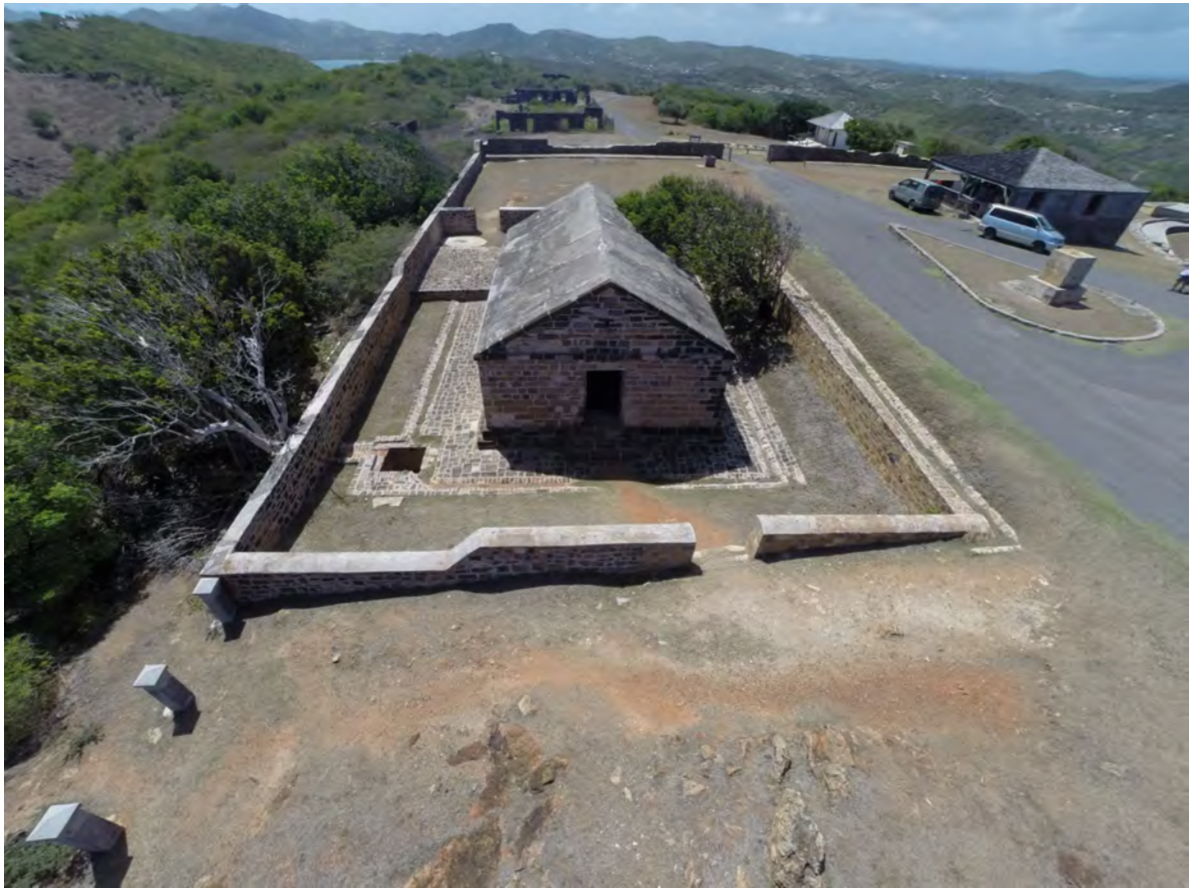
Figure 65. Ariel view of Blockhouse Powder Magazine with Ruins of Officers Quarters in the back ground.
