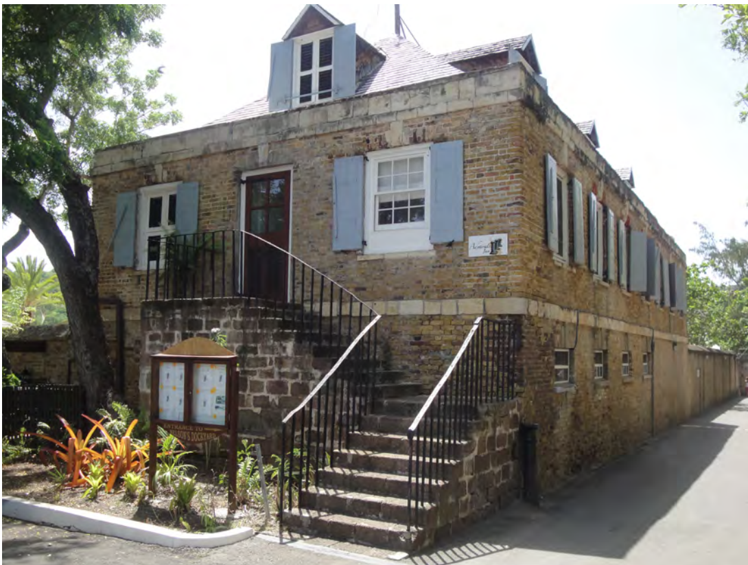
Figure 17. The Engineers House West elevation
