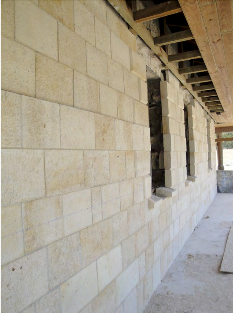
New stonework façade on upper floor exterior.
