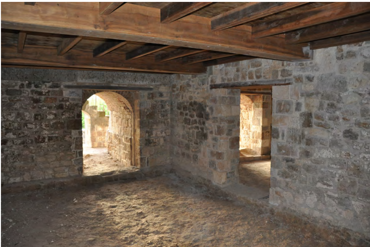
Figure 76. Greenheart beams and joists of main floor seen from lower level.
