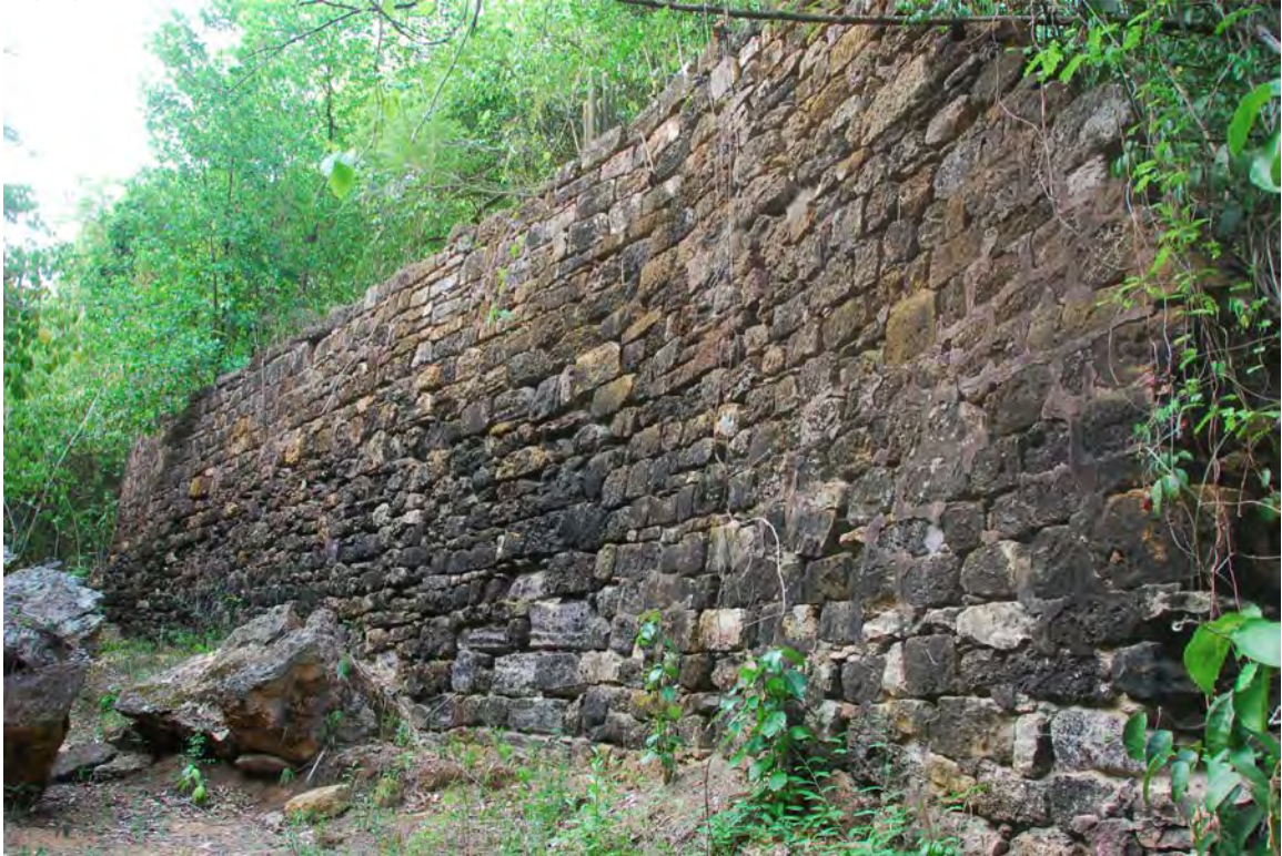
Figure 40. End wall of dam at Jones Valley.
