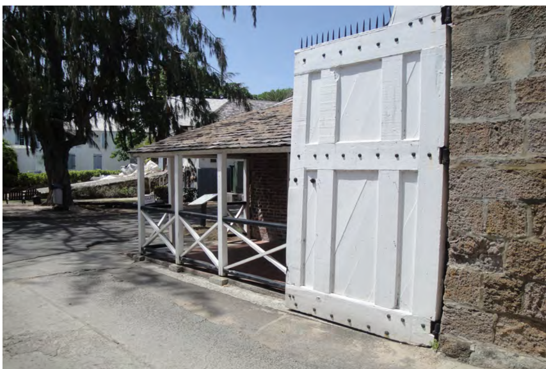
Figure 132. Entry gate and Gate house.
