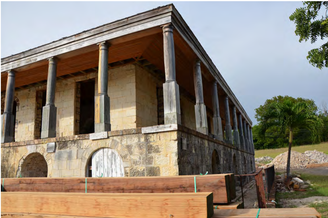
Figure 112. Clarence House Restoration.
