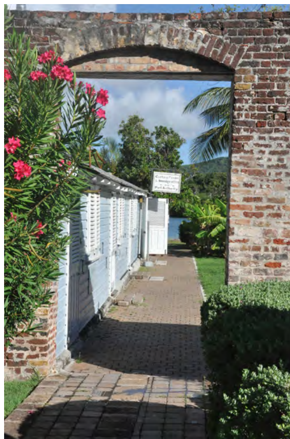
Figure 28. Remaining Walls of Canvas and Cordage Building
