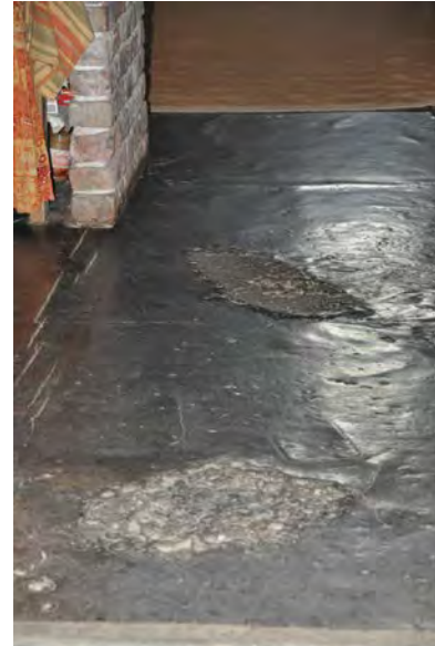
Figure 62. Pitch floor in Powder Magazine
