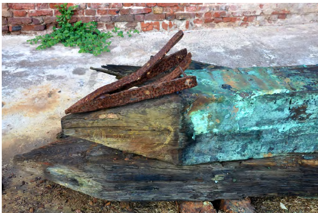
Figure 44. Original Piles sheathed in copper
