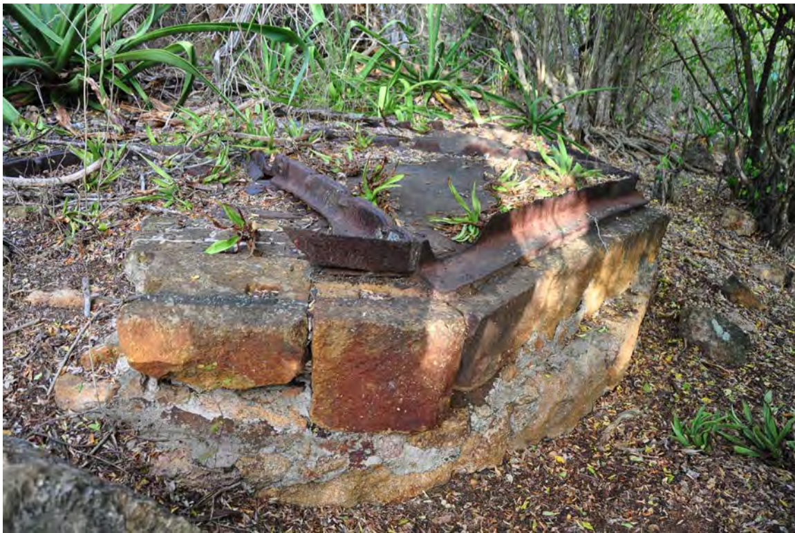
Figure 39. Base and bottom of cast iron water tank.
