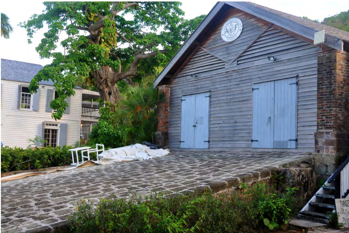
Figure 37. Ramp up to the saw Pit Shed
