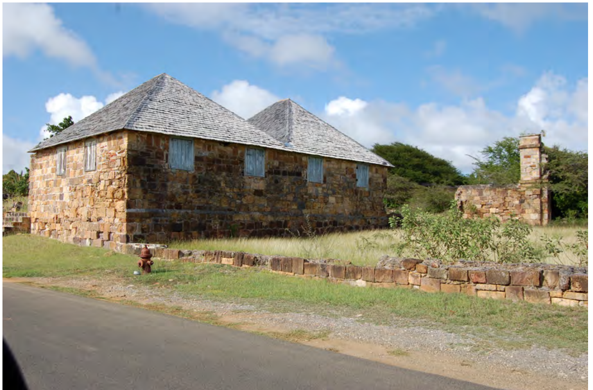
Figure 66. Store rooms for the Artillery Complex now used as the Archaeological research center.
