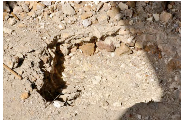
Test hole dug in verandah floor near main front entrance.
