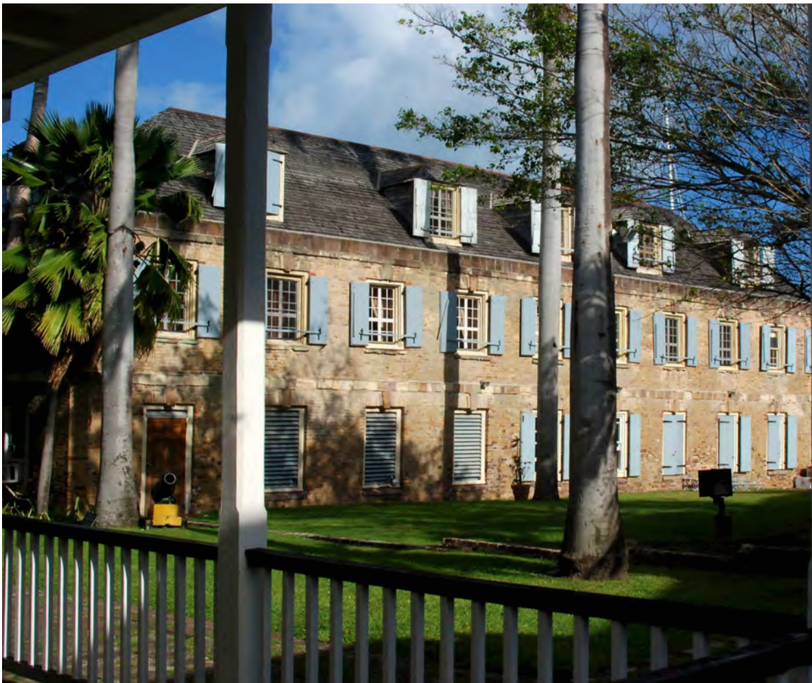
Figure 134. Copper & Lumber Store south elevation.
