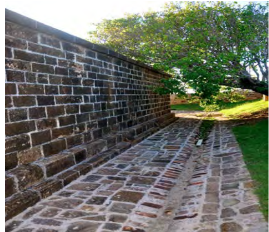
Figure 6. Water collection Blockhouse.
