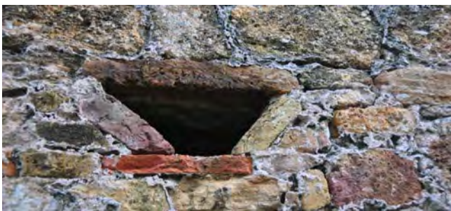
Figure 23. Stone wall detail, Artillery Complex.
