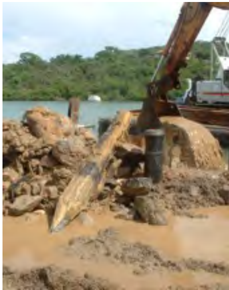
A wooden pile emerges, then the copper clad wall.
