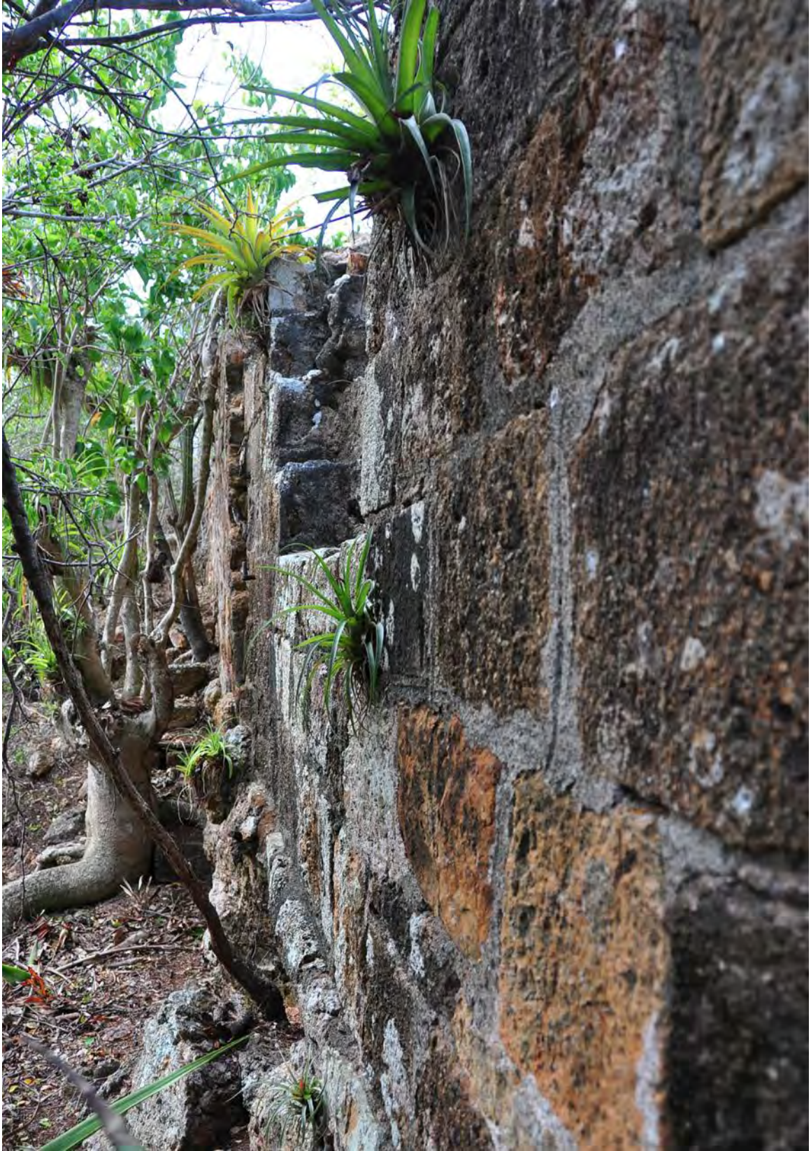
Figure 37. Exterior wall of ruined structure on north side of the Ridge.
