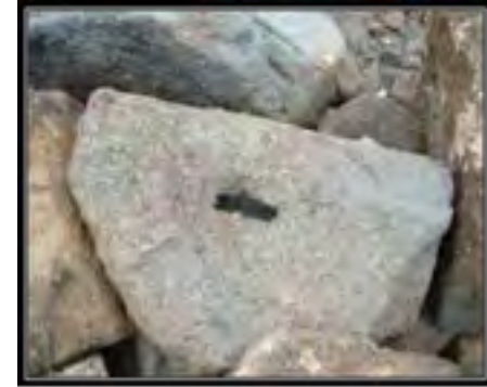
This tool known as a Lewis fitted into the dovetail cut in the rock. It could then be lifted.
