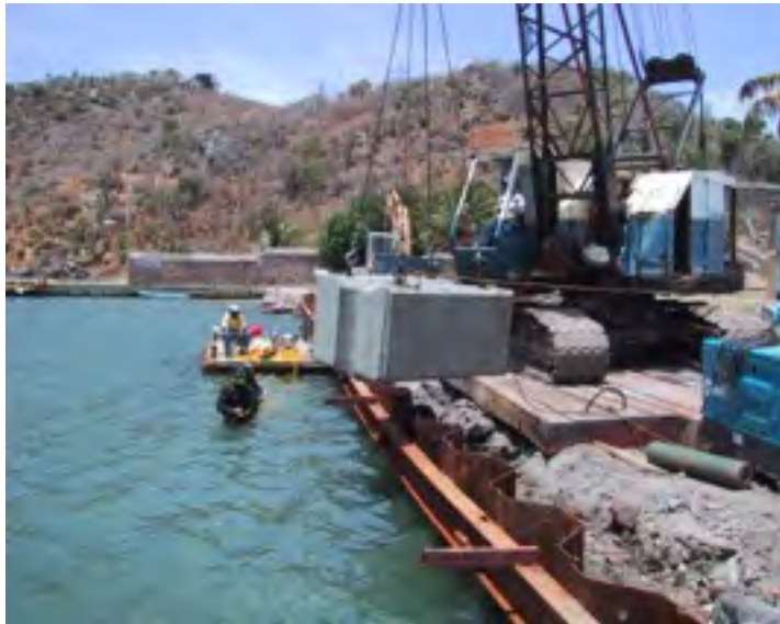
Placing the interlocking blocks.
