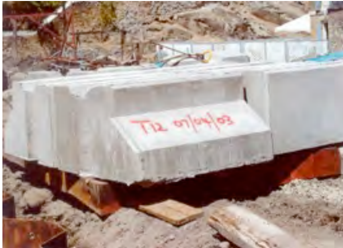
Concrete blocks for the base of new wall.
