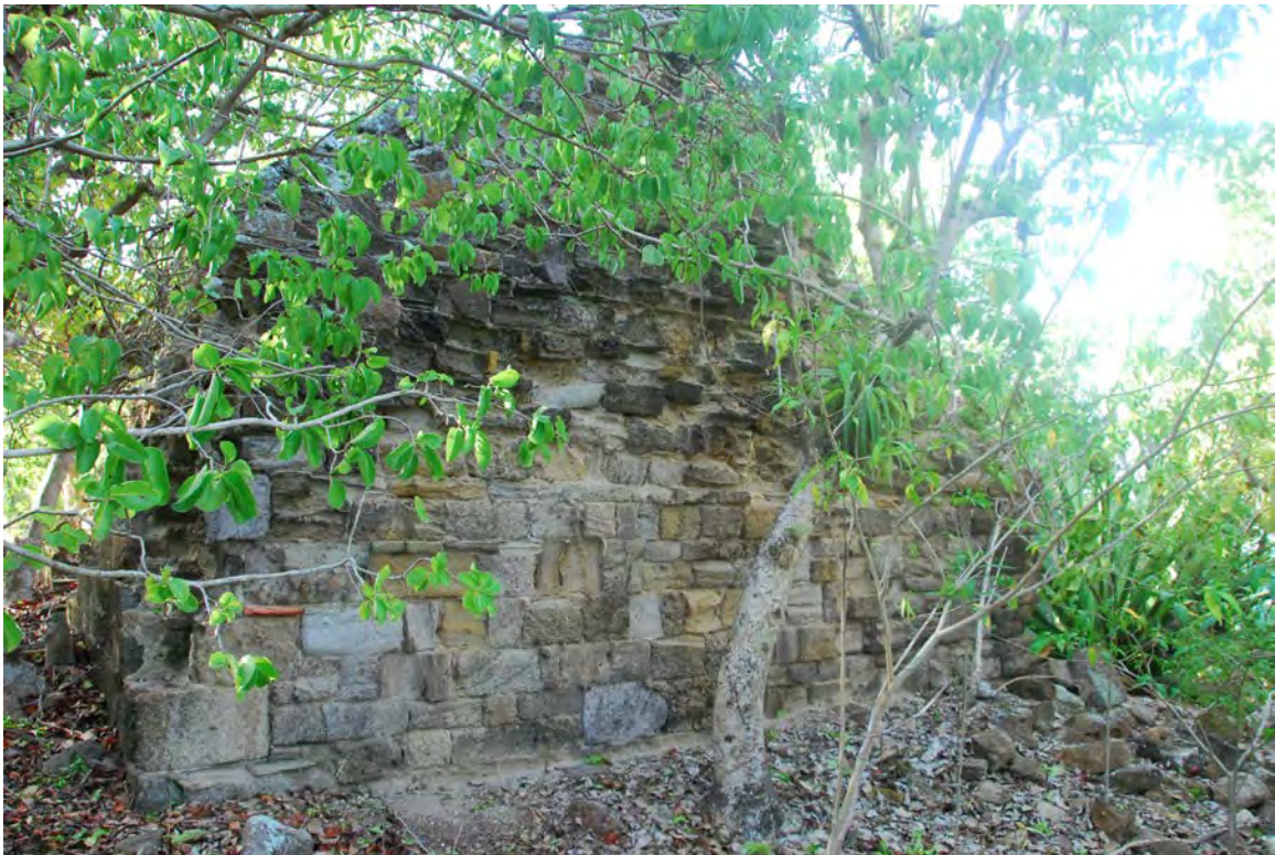
Figure 20. Gable end wall possibly of Kitchen.
