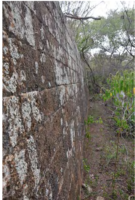
Figure 32. North wall Dow's Hill Bastion also in good repair.
