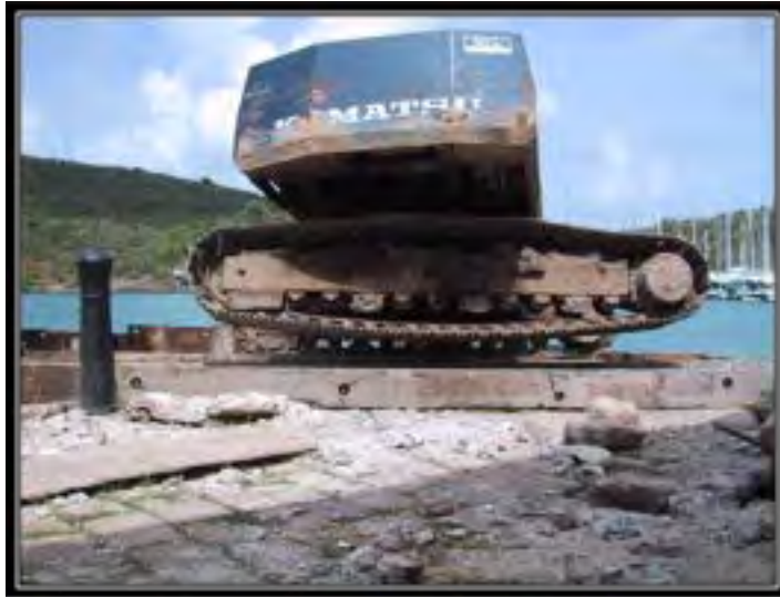
Lifting the largest stones was at times challenging.
