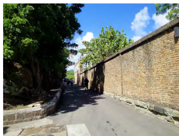
Figure 40. Brick Wall enclosing compound
