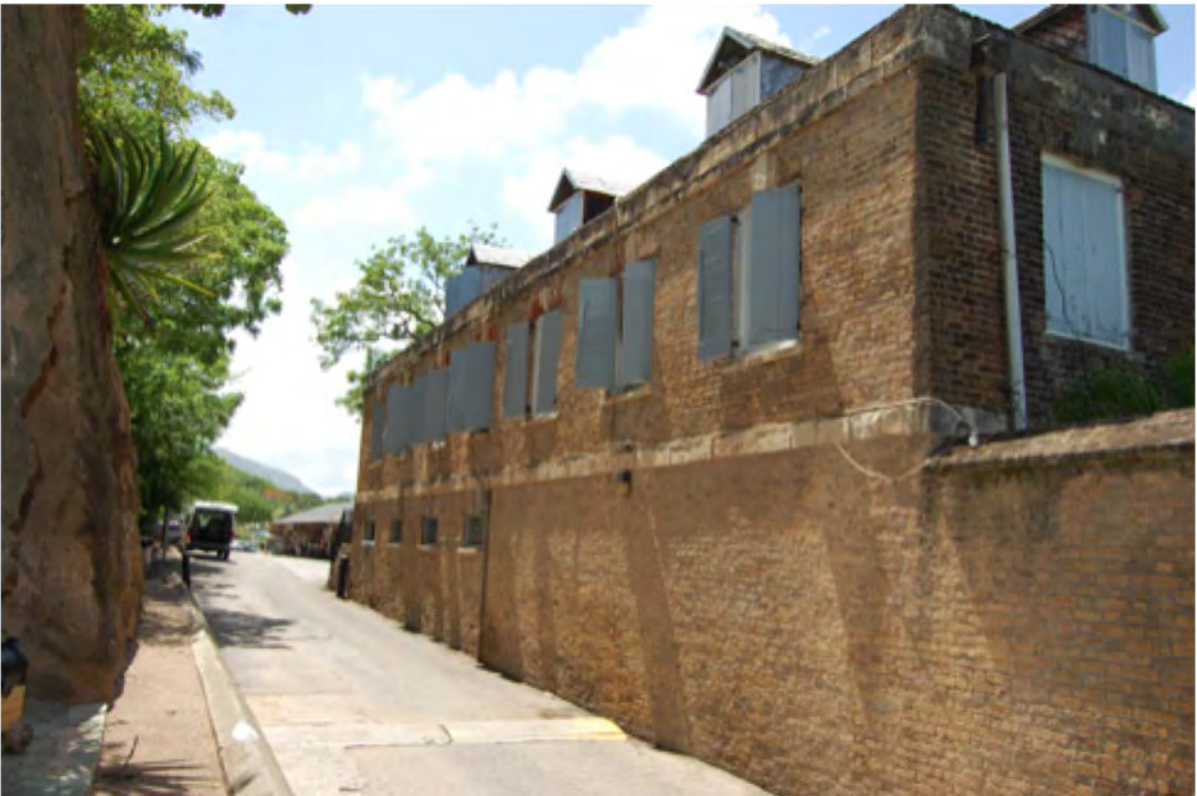
South elevation Engineers Building and entry road to the Dockyard
