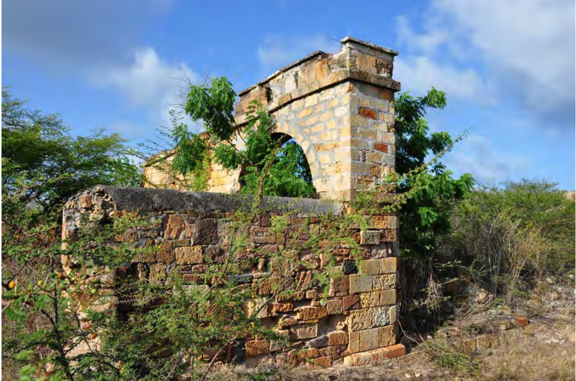
Figure 22. Original stone arch with added on stone wall.
