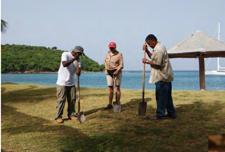
Day 1. Removal of sod.
