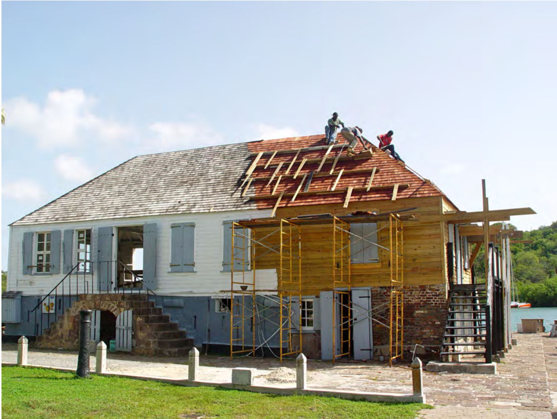
Figure 111. The Pay Office having major repairs done to the woodwork.
