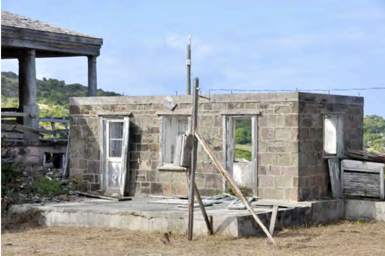
Clarence House kitchen (demolish and rebuild elsewhere).
