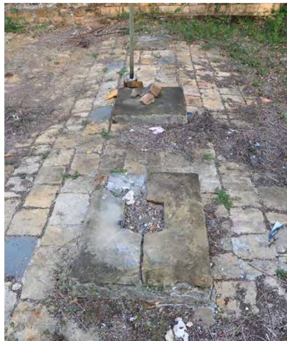
Figure 63. Stone floor and Column bases, remains of storage area.
