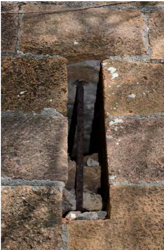
Figure 31. Detail, west wall Dow's Hill Bastion, in good repair.
